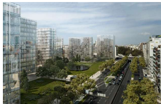
"ENTRECAMPOS" project — Lisbon, Portugal
