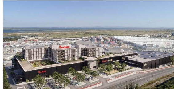
Alverca shopping centre transformation project — Portugal
