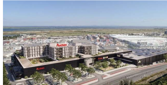
Alverca shopping centre transformation project — Portugal
